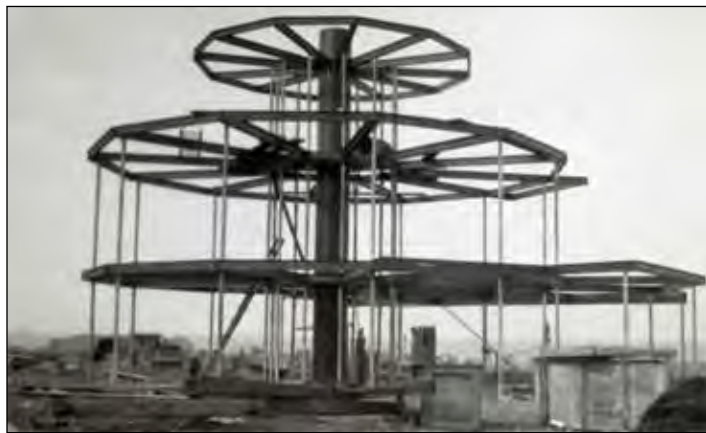
The steel framework of the House of Tomorrow.
